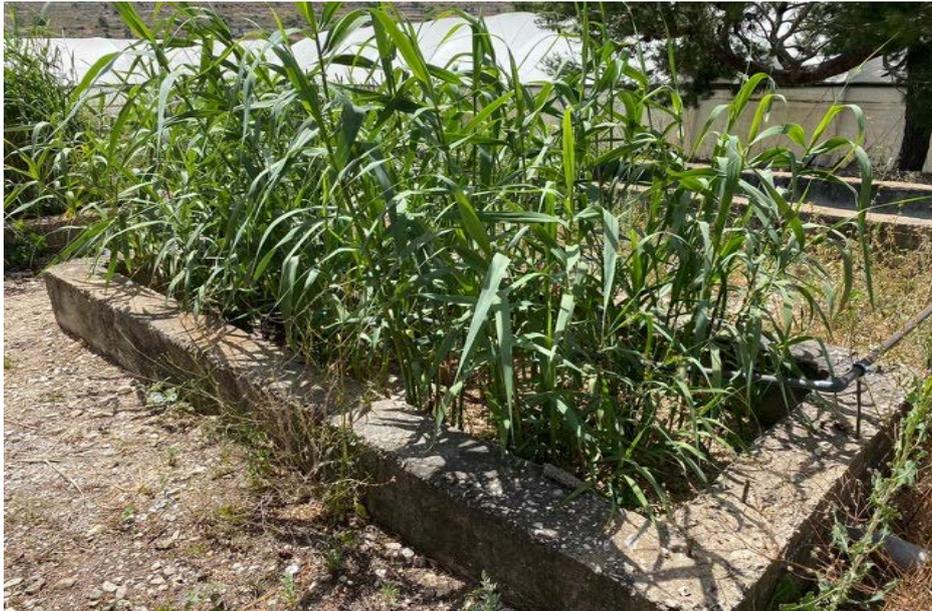
Photo of the constructed wetland basin cultivated with common reeds
