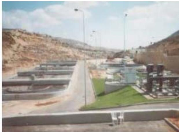
Photo 5: Al-Bireh extended aeration system for wastewater treatment
