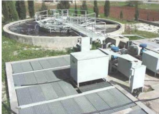
Photo 4: Birzeit water recovery facility through contact stabilization system
