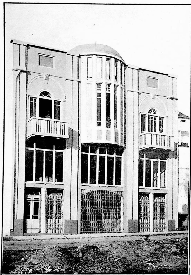
SHOPS AND OFFICES AT TEL AVIV BUILT OF CONCRETE AND CEMENT BRICKS BY THE JEWISH CO-OPERATIVE LABOUR ASSOCIATION.
