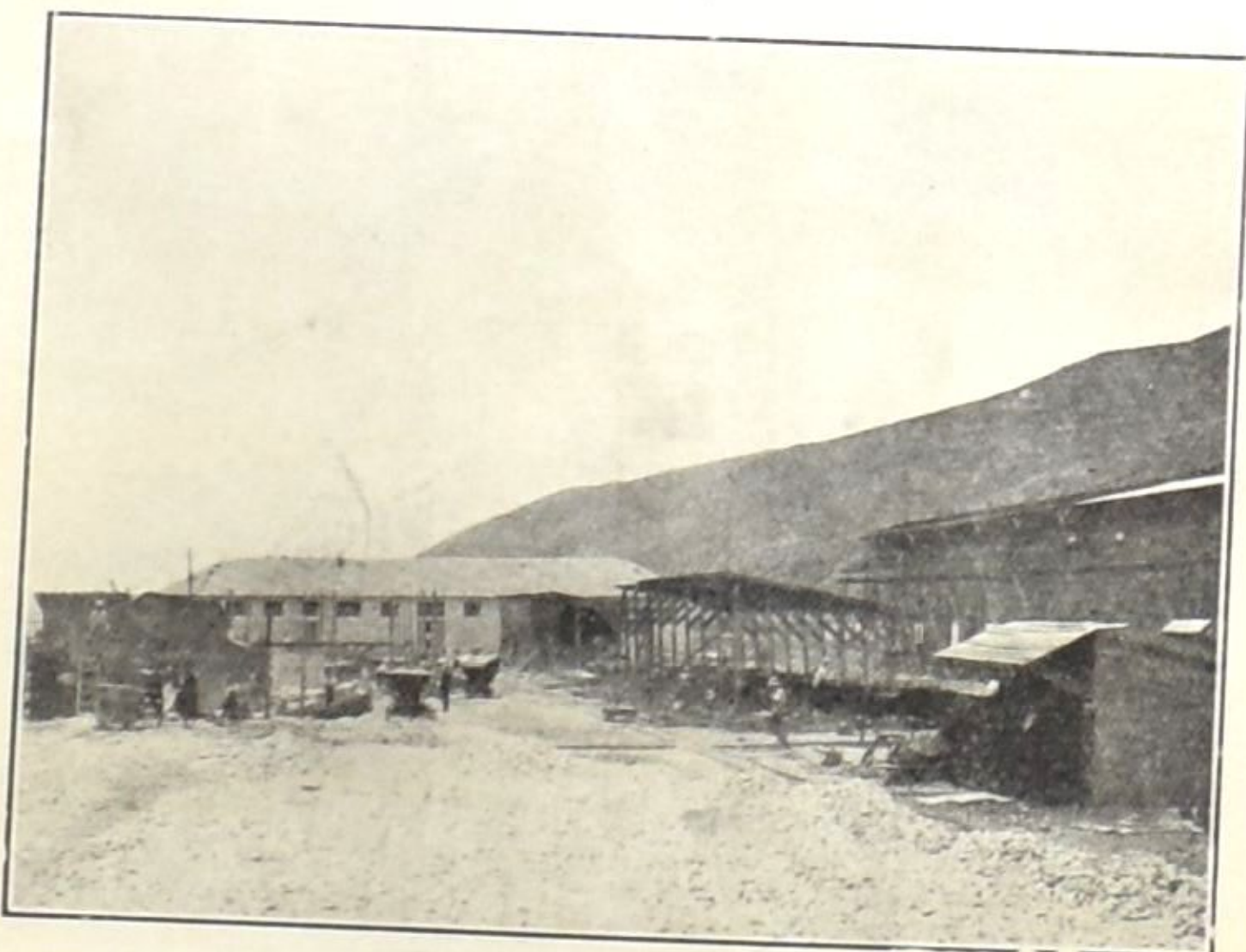
HILL, FROM WHICH RAW MATERIAL FOR THE MANUFACTURE OF CEMENT IS OBTAINED. [Photo by P. W. Etkes.]
