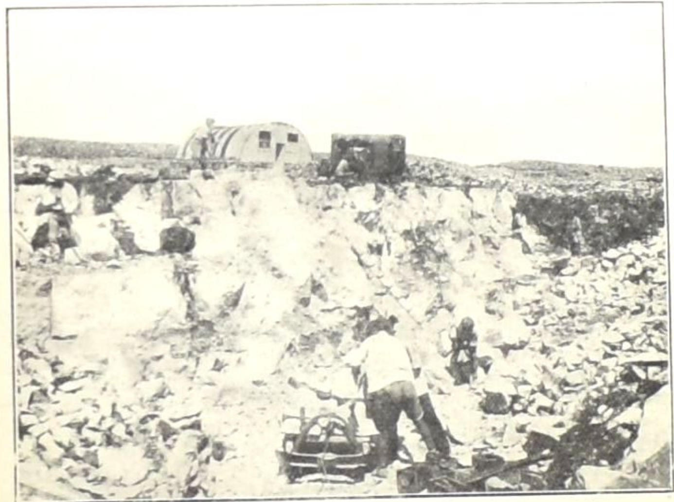
STONE QUARRYING BY MEANS OF COMPRESSED-AIR DRILLS AT JERUSALEM BY SOLEL BONEH ORGANISATION.
