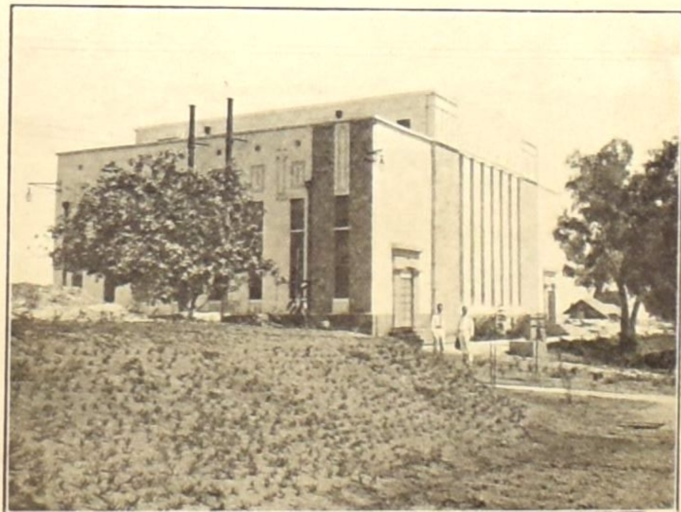
POWER STATION OF THE PALESTINE ELECTRICAL CORPORATION UNDER THE RUTENBERG CONCESSION.
