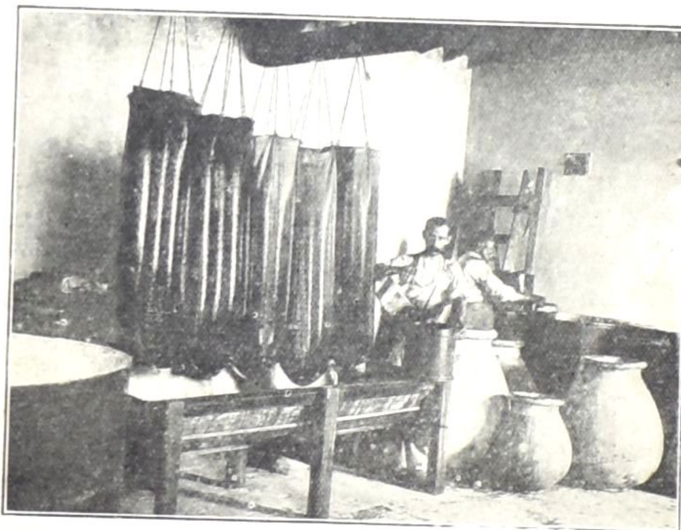
[Photo by Mr. Struve, Junr.] FILTRATION AND STORING OF SESAME OIL, AT FACTORY OF MESSRS. STRUVE AND CO.
