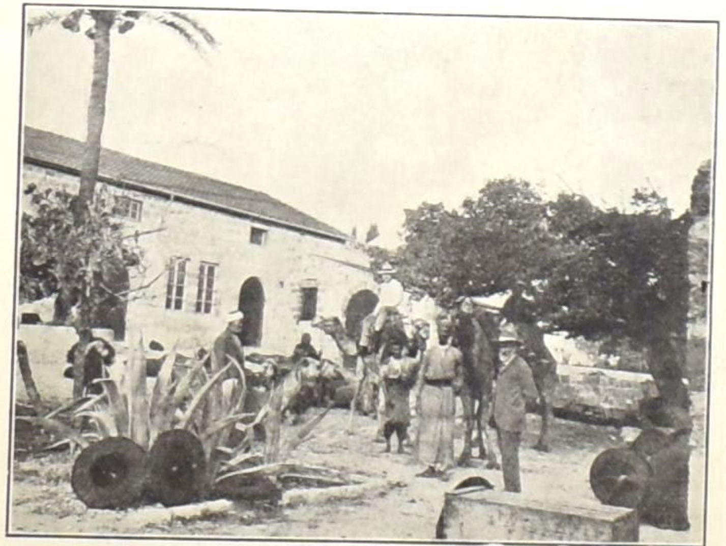
SESAME OIL AND SOAP FACTORY OF MESSRS. STRUVE AND CO. IN HAIFA. [Photo by Mr. Struve, Junr.]
