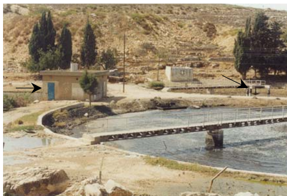
FIGURE 3a. Operation room and tow aerated ponds (aerator out of operation in background) of RWWTP
