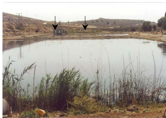
FIGURE 3b. Two polishing ponds (chlorinating unit and a by-pass road of an Israeli colony, background)
