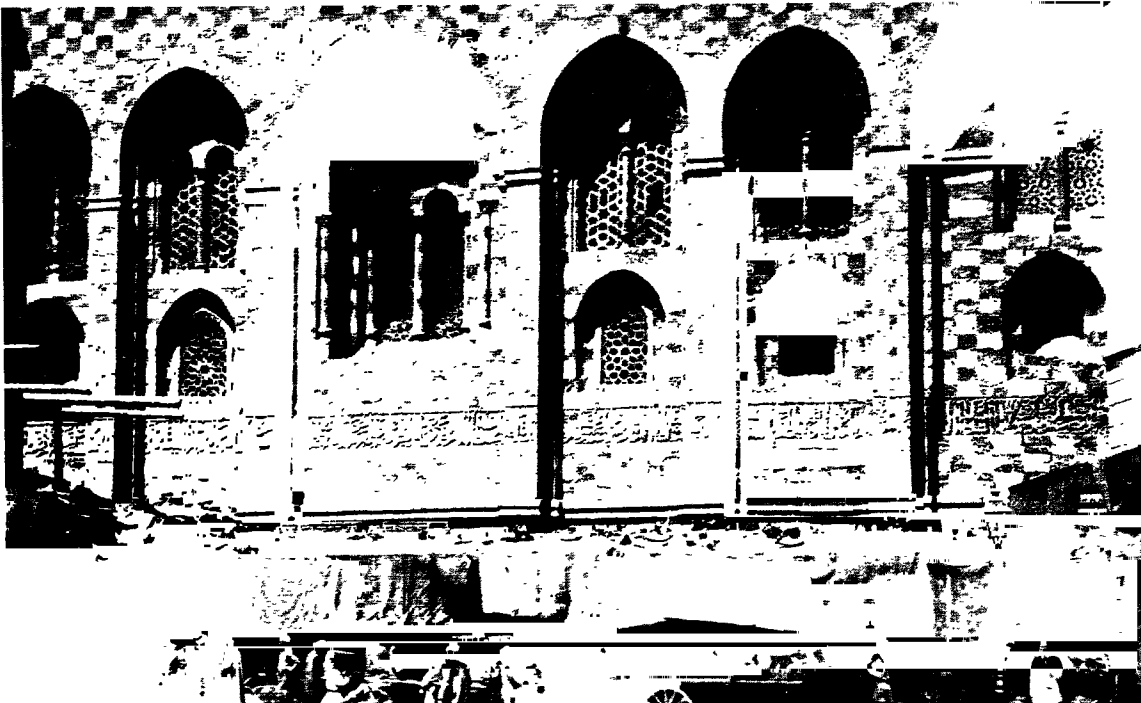
FIG. 62. CAIRO : MAUSOLEUM OF QALĀWŪN. Exterior before restoration
