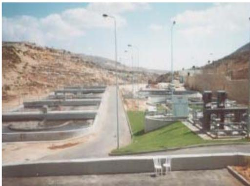
Photo 5: Wastewater treatment plant/ extended aeration system/ Al-Bireh City/ the West Bank / Palestine
