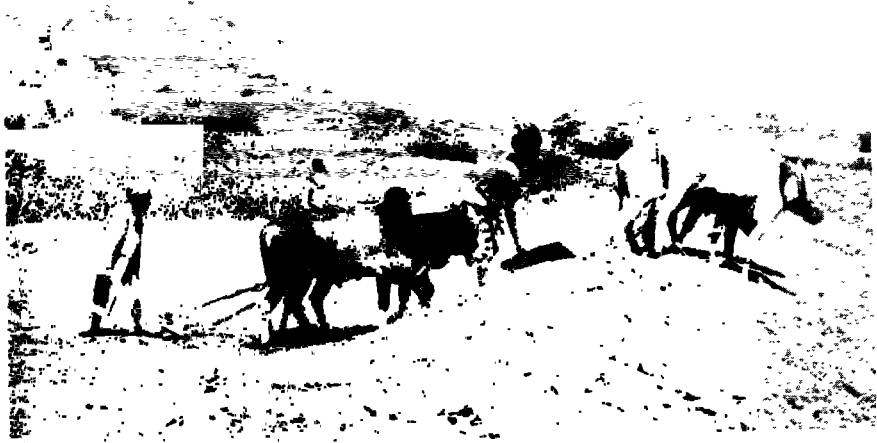
243. Building earthen dikes before irrigation at Dhāla'
