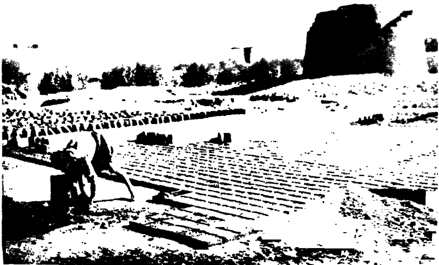
272. Drying bricks in the sun, San'a
