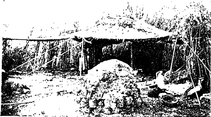
FIG. 3.—Bedawy tent. A mere roof with some stalks round it on the windward side. In Syria, flaps of camel-hair cloth are hung to windward. (p. 14.)
