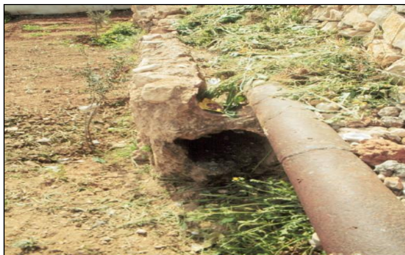
Figure 11. Installed iron water pipe during the Ottoman epoch. From [10].
