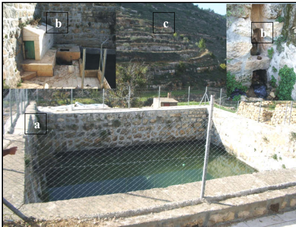
Picture 4: 'Ein Jami' spring and its collection pool (a), water delivery system (b), and the surrounding terraces (c).
