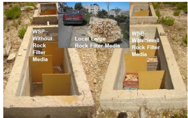
Fig. 2. Overview of the upgraded systems (wooden baffles and biofilter in ARPs) (photos courtesy of Maher Abu-Madi and Omar Zimmo)
