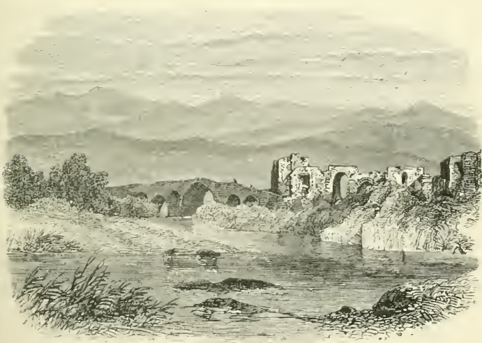
BRIDGE OVER JORDAN.
