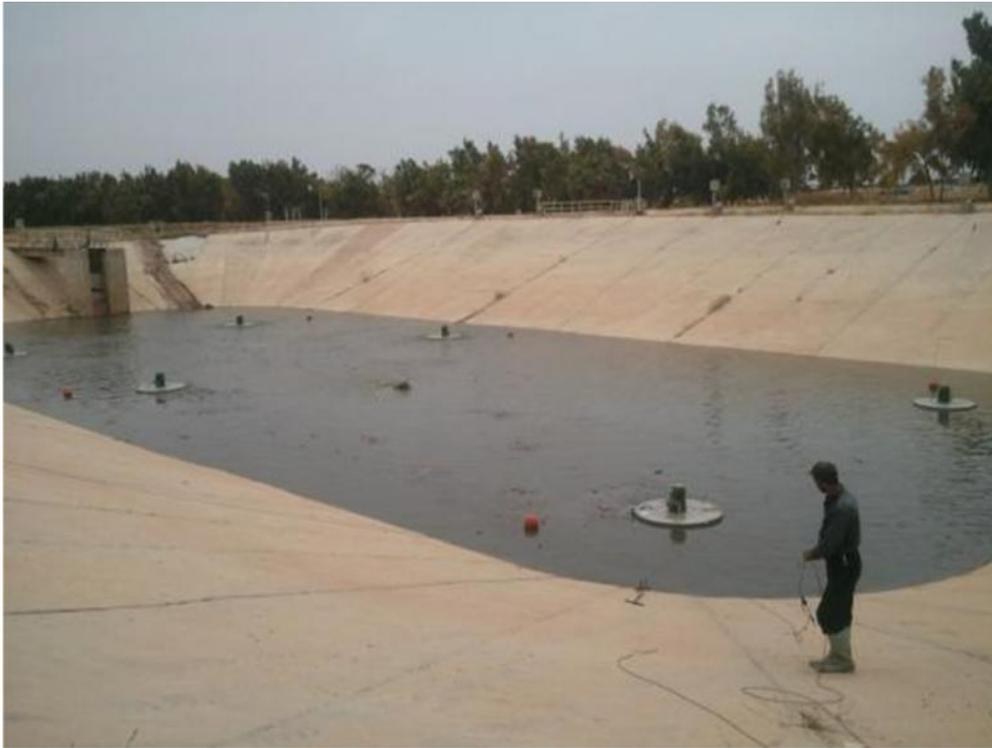
Figure 8: Preparation of the equalization tank
