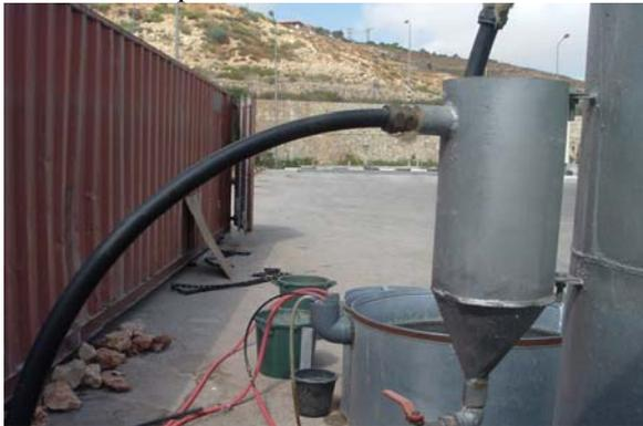
**Photo A.3.** Connecting container which collect the UASB-septic tank effluent. The photo shows also the hose which convey the effluent to the holding tank (see photo A.4).
