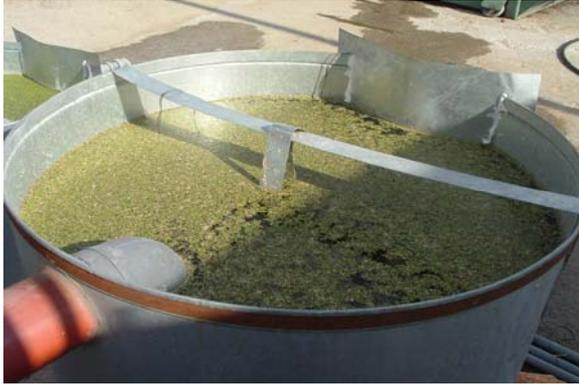
**Photo A.7.** Galvanized steel holder for the sedimentation cup, two rods were used for the purpose of holding; the first rod (vertical) was used to hold the cup and keep it from turn over and the second one (horizontal) was used connect the vertical holder on the pond body.
