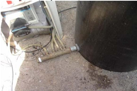
**Photo A.5.** Suction point from the holding tank by the pumps to the stabilization ponds. The MASTER FLEX hoses are also shown. The photo shows also the pump feeding the deepest stabilization ponds.
