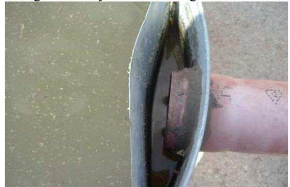
**Photo A.6.** The baffle which was installed for preventing short circuiting of wastewater and to prevent floating materials from transporting to successive stabilization ponds. The 4" PVC pipe connecting stabilization ponds is also shown
