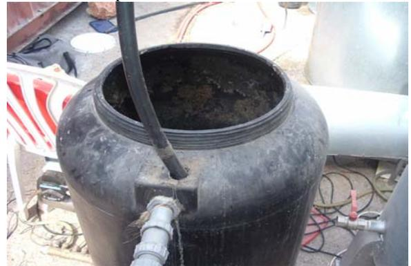
**Photo A.4.** Holding tank, (collection reservoir for the UASBs' effluent). The photo shows also the overflow line from which excess pretreated sewage is conveyed back to the grit chamber.
