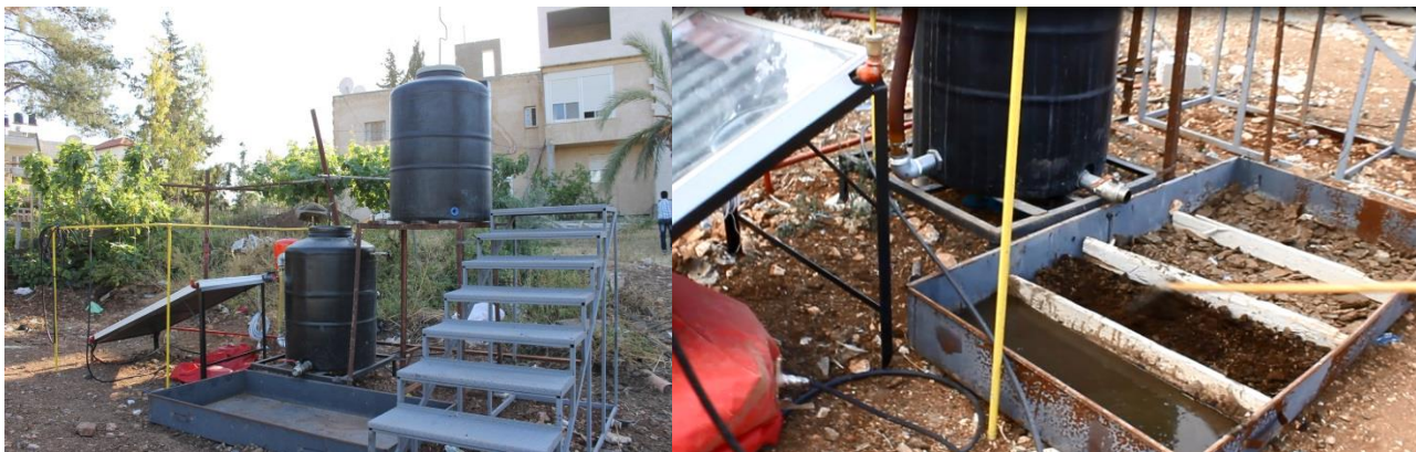
a. A waste collector tub as a part of plant design
