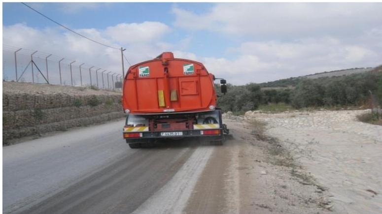
**Figure 3.10: Control on dust**
