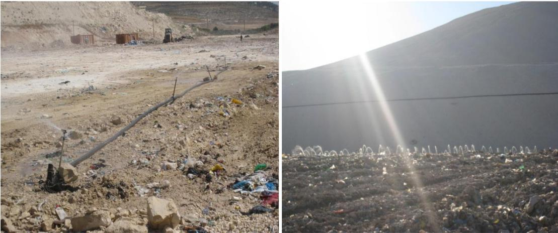
**Figure 3.15: Recycling leachate and evaporation**
