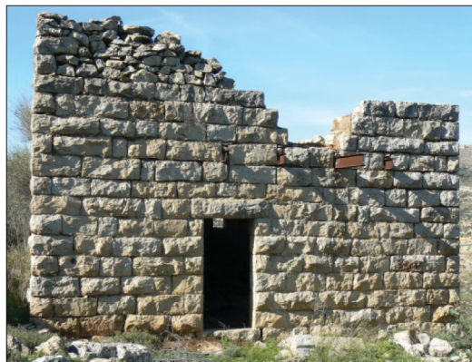
Figure 13. Drawings and a photograph showing a watchtower with a flat ceiling constructed of iron I-beams and cement: a) plan, elevation and section for a quadrilateral watchtower, with dressed ashlar stone and mortar and b) front view, with main entrance. Note the protruding iron beams, which probably supported a small upper-level balcony (color figure available online).
