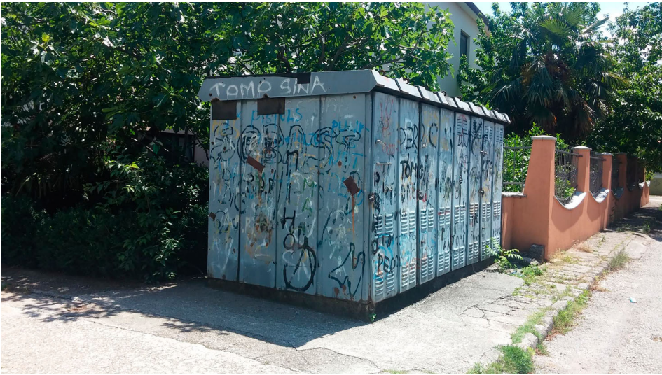
Figure 2. The transformation of an electric substation into the monument dedicated to the miners (Marko Barišić, 2016).
