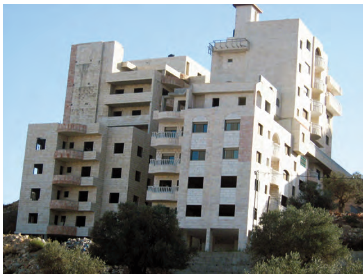
Figure 8. A new private housing project built in Ramallah city after 2000, using an informal cooperative approach.
