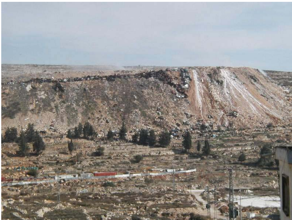
Photo No. 2: Ramallah Dumpsite: reaching a 60 m height
