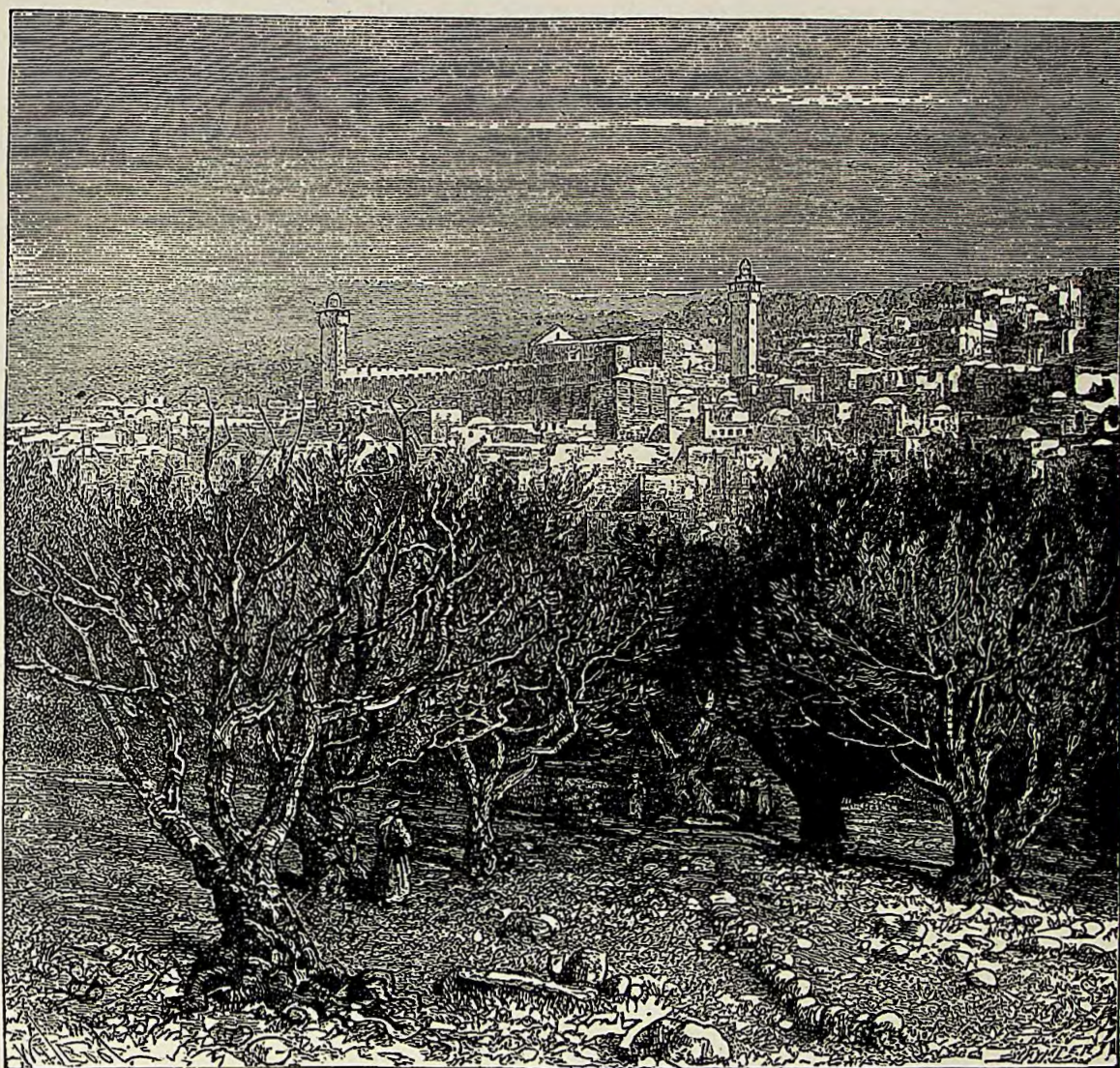
HEBRON, AND MOSQUE OVER THE CAVE OF MACHPELAH.
