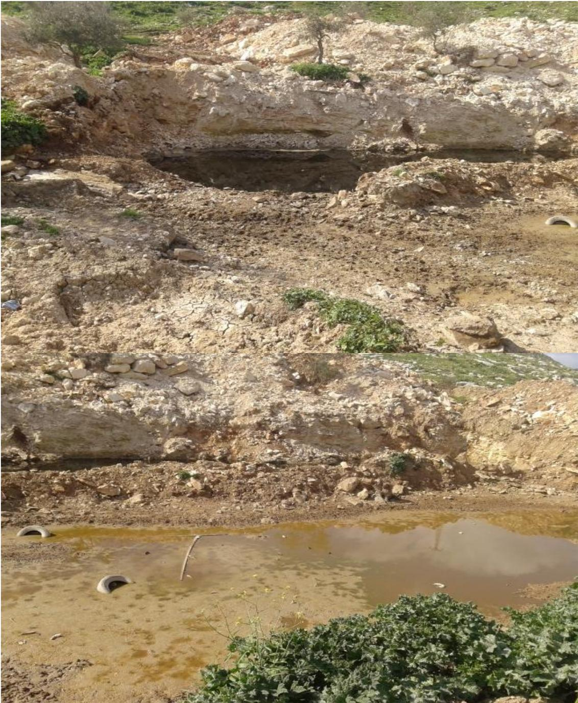
Figure 3.6: Leachate accumulation outside the landfill
