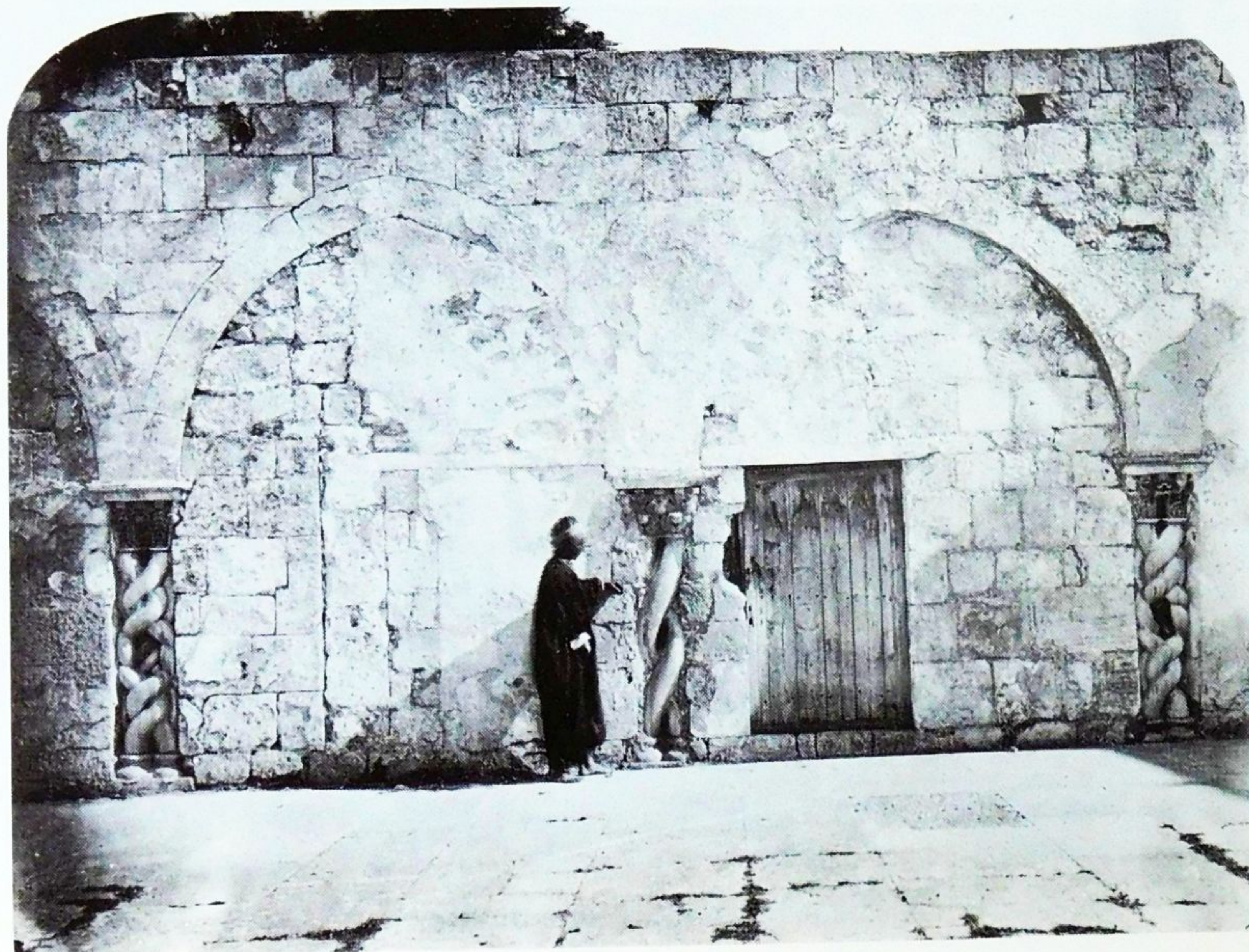
5b. S. W. CORNER OF THE PLATFORM
