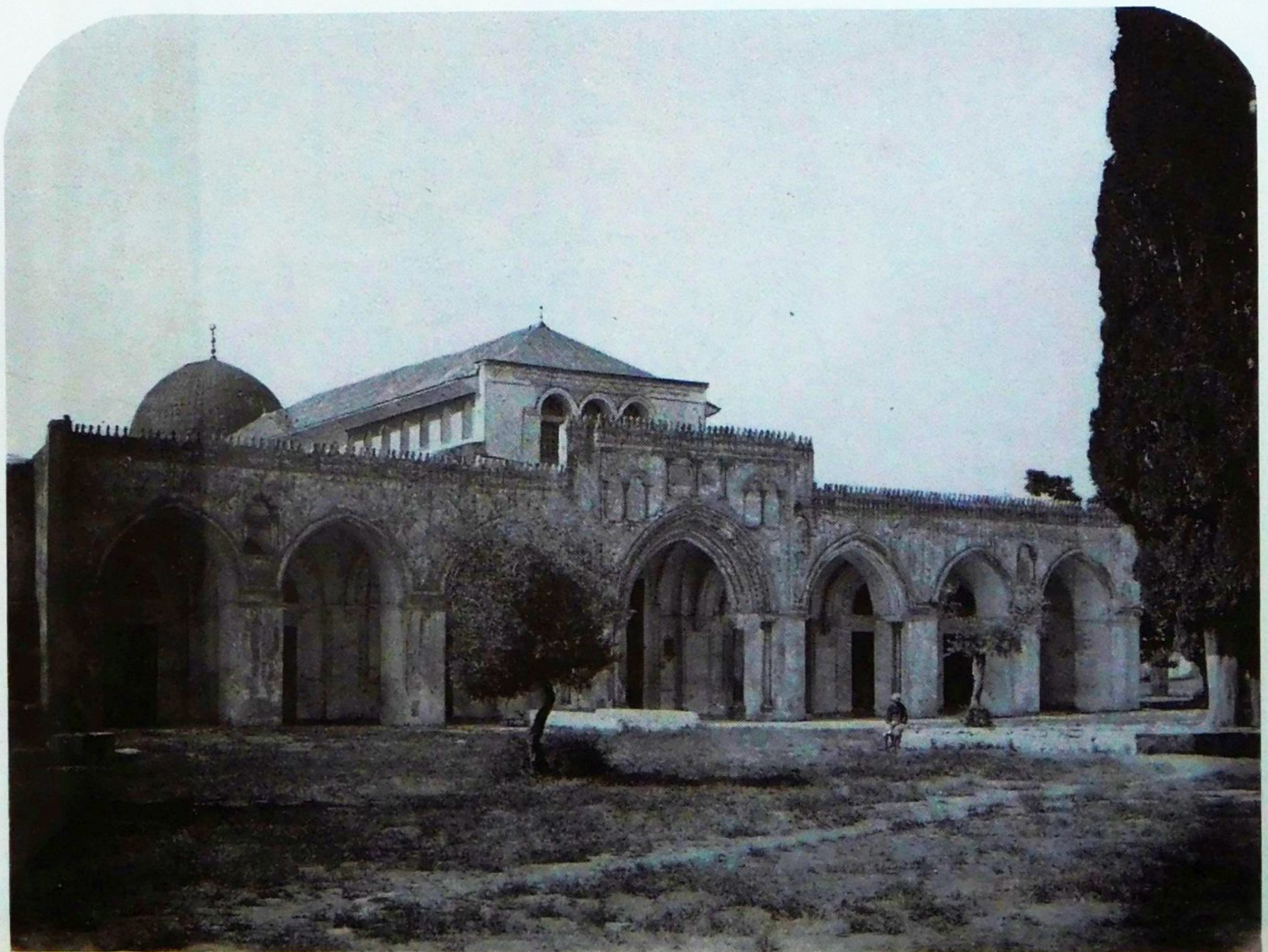
8b. NORTH FRONT OF MASJED AL AKSA
