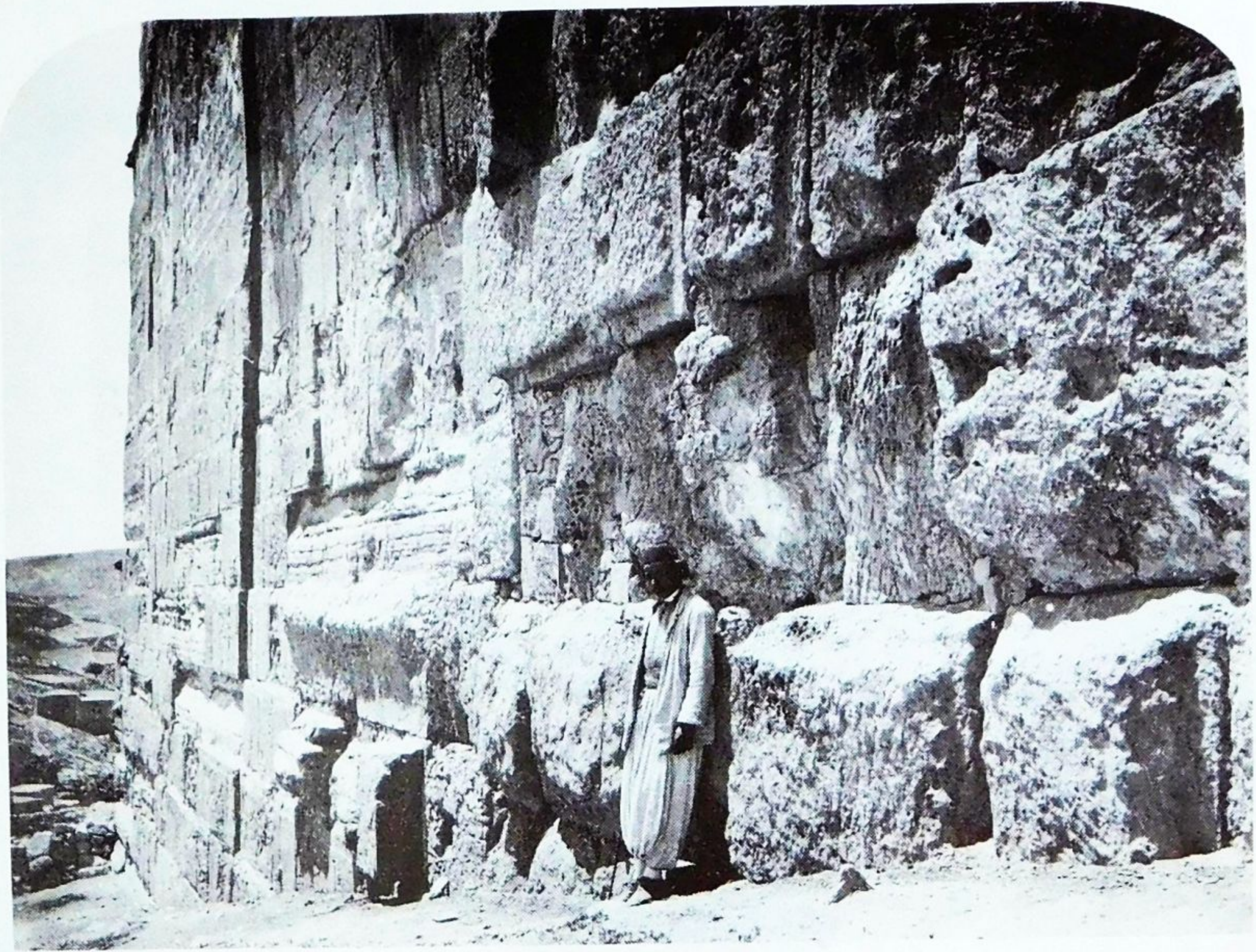
11a. EASTERN WALL NEAR SOUTH-EAST ANGLE
