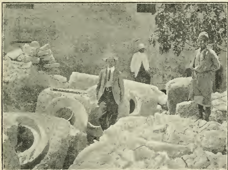
FIG. 1.—Disjointed Tubes of the Stone Syphon.
