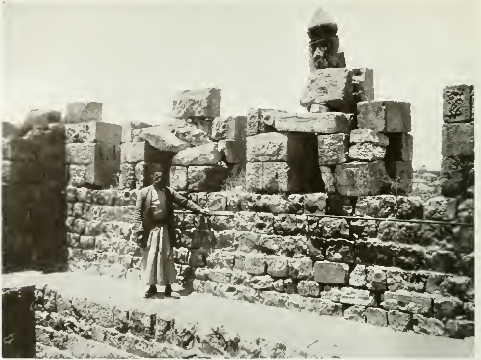
Damascus Gate pinnacles before repair.
