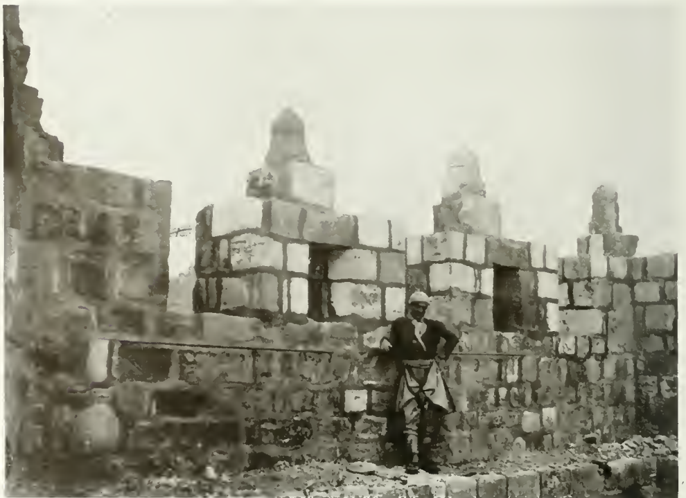
Damascus Gate pinnacles after repair.
