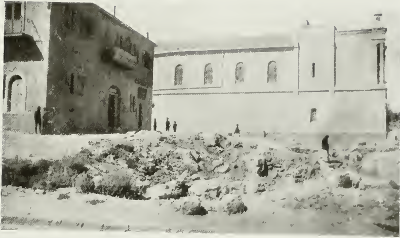
Post Office Square, before treatment.
