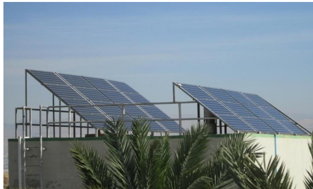
Figure 19: Photo of the PV arrays in Al- Zubiedat BWRO dealinatio unit, (Yousef, 2013)
