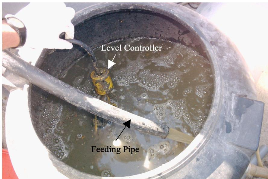
**Photo 6.** The photo shows the level controller device that was used to control the wastewater level inside the holding tank. In addition to the raw sewage feeding pipe that comes from the grit removal chamber at Al-Bireh WWTP
