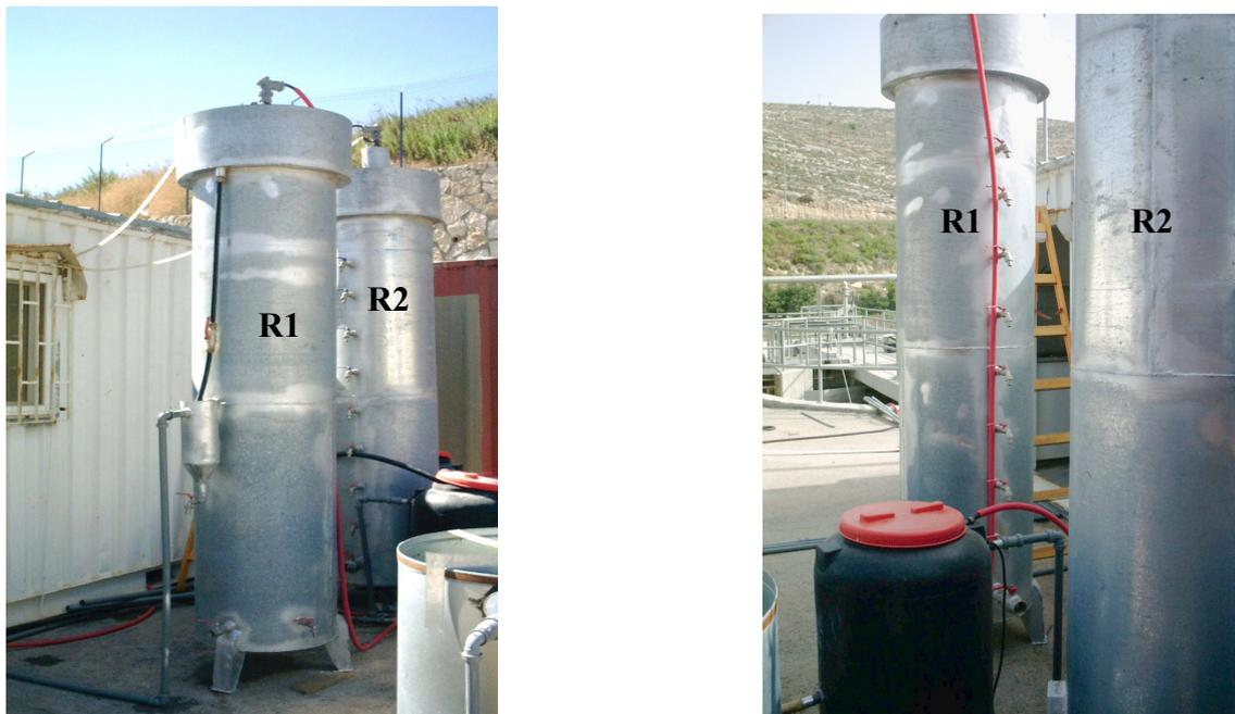
**Photo 2.** Side view of the UASB-septic tank reactors (R1&R2) and the holding tank from which the reactors were fed
