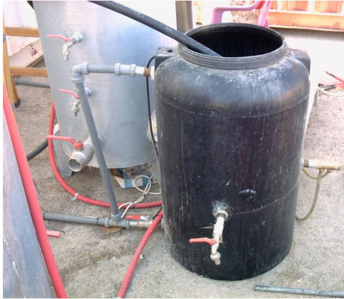
**Photo 5.** The holding tank that was used for feeding the two pilot UASB-septic tank reactors. The photo also showing the overflow and the recirculation pipes of the holding tank.
