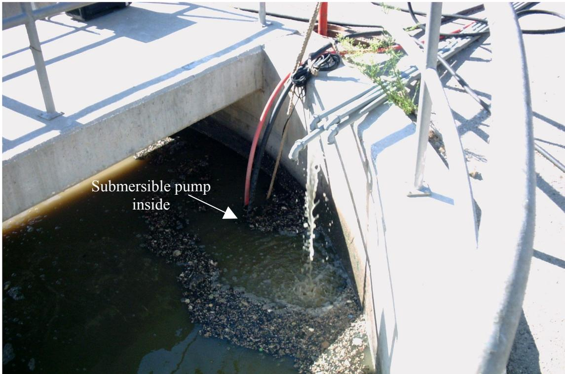
**Photo 8.** The grit removal chamber at Al-Bireh WWTP that from which the raw sewage was fed to the pilot plants. The photo also shows the pipes used to return sewage from the holding tank and the effluents of the pilot plants
