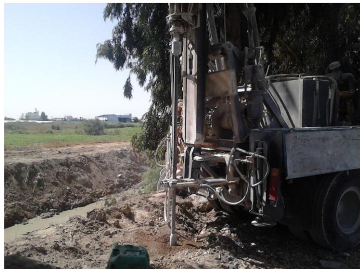
**Figure 3.5:** Borehole drilling closed to Wadi Al Zomar using mobile rig machine
