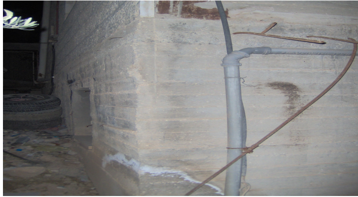
Photo 9. Separation system for kitchen sink
