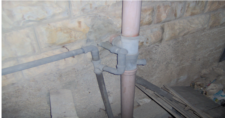
Photo 6. Separation system for toilet, kitchen sink and shower +hand basin effluent domestic household Wastewater for several houses
