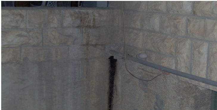
Photo 7. Separation system for kitchen sink
